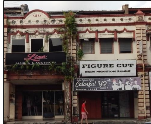
Figure 6: Palladian design shophouse
