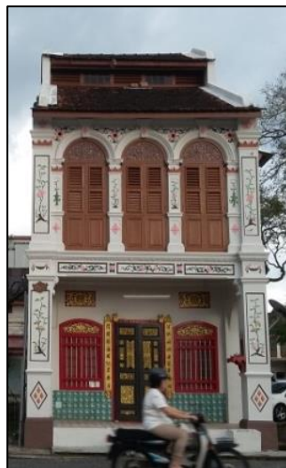
Figure 8: Double roofing of shophouse in Taiping.
